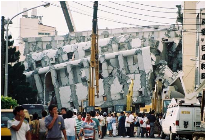
Fig.1 Street blocked by a fallen building
